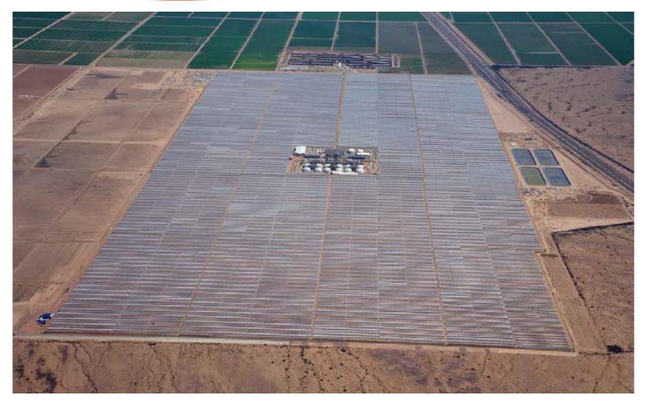
Power Block and TES is located at the center of the solar field
