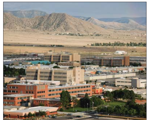
Sandia National Laboratories/ New Mexico Water Consumption Reduction
