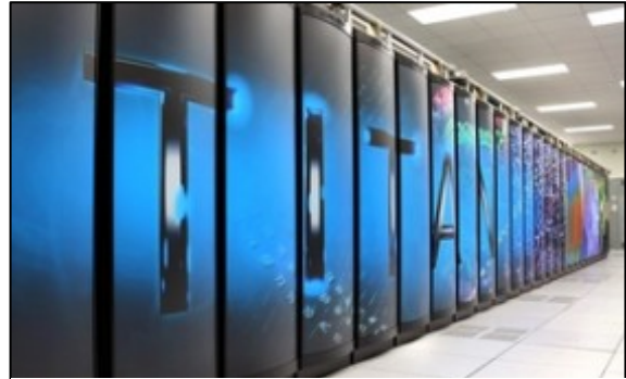
ORNL's TITAN Supercomputer
