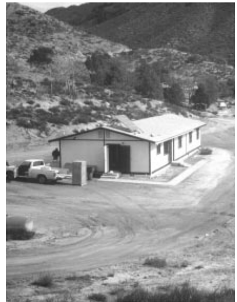
LOS COYOTES TRIBAL HALL IS EQUIPPED WITH SOLAR PANELS.
