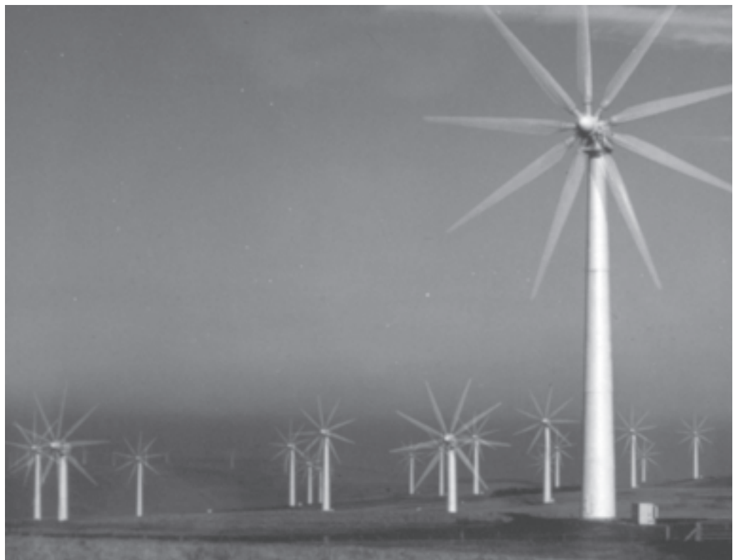
A COMMERCIAL WIND GENERATION FACILITY IN PALM SPRINGS, CALIFORNIA.
