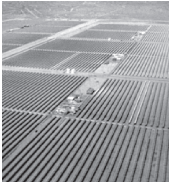
ABOVE: A SOLAR THERMAL LINE-CONCENTRATOR SYSTEM OPERATED BY KSC OPERATING CO. PROVIDES POWER TO SOUTHERN CALIFORNIA EDISON COMPANY. (PHOTO: ELECTRIC POWER RESEARCH INSTITUTE) RIGHT: THE CENTRAL RECEIVER CONCEPT WAS SUCCESSFULLY DEMONSTRATED AT THIS DOE-SPONSORED 10-MW PILOT PROJECT, CALLED SOLAR ONE, LOCATED IN BARSTOW, CALIFORNIA. (PHOTO: MCDONNELL DOUGLAS)
