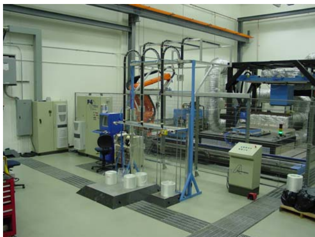
Figure 2. Fiber delivery system and operating controls for ORNL's preforming system.
