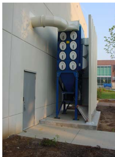
Figure 3. External filter system for ORNL's preforming system.
