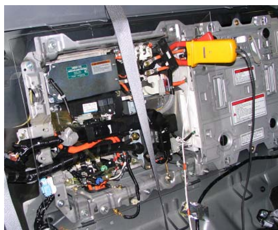
Figure 1. Accord HEV battery and electronics bay behind rear seat
