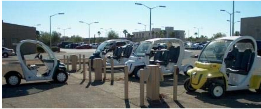
Figure 2. Luke Air Force Base NEVs Charging at 110 Volts
