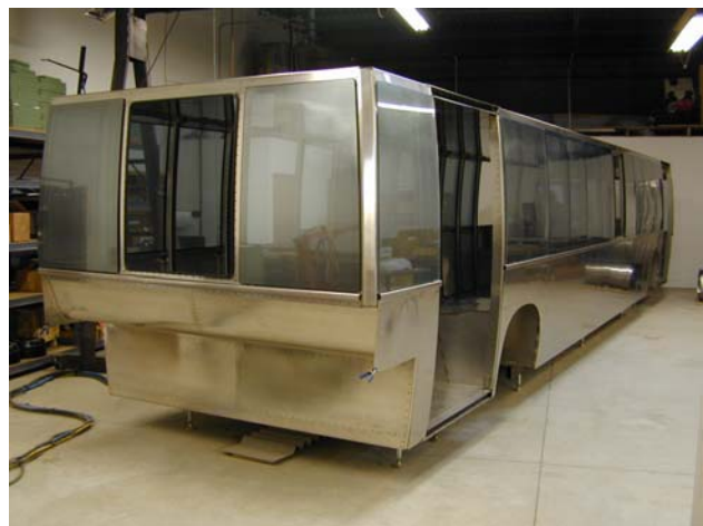
Figure 1. Installation of side and rear windows
