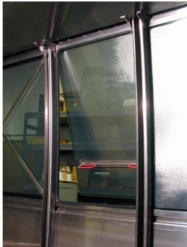
Figure 4. Installed emergency exit window
