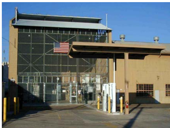
Figure 1. APS Alternative Fuel (Hydrogen) Pilot Plant, with fuel dispensing island in the foreground.
