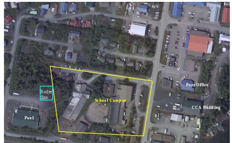
Craig, AK – Wood chip district heating system
