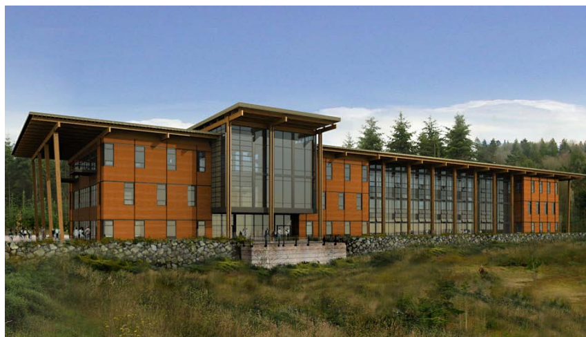
Tulalip new Administration Building uses geothermal generated power
