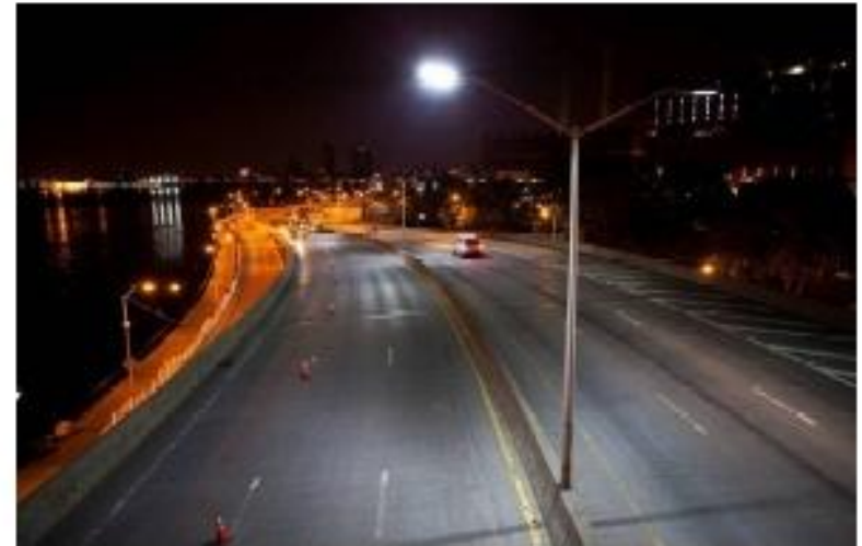
FDR Expressway, NYC
