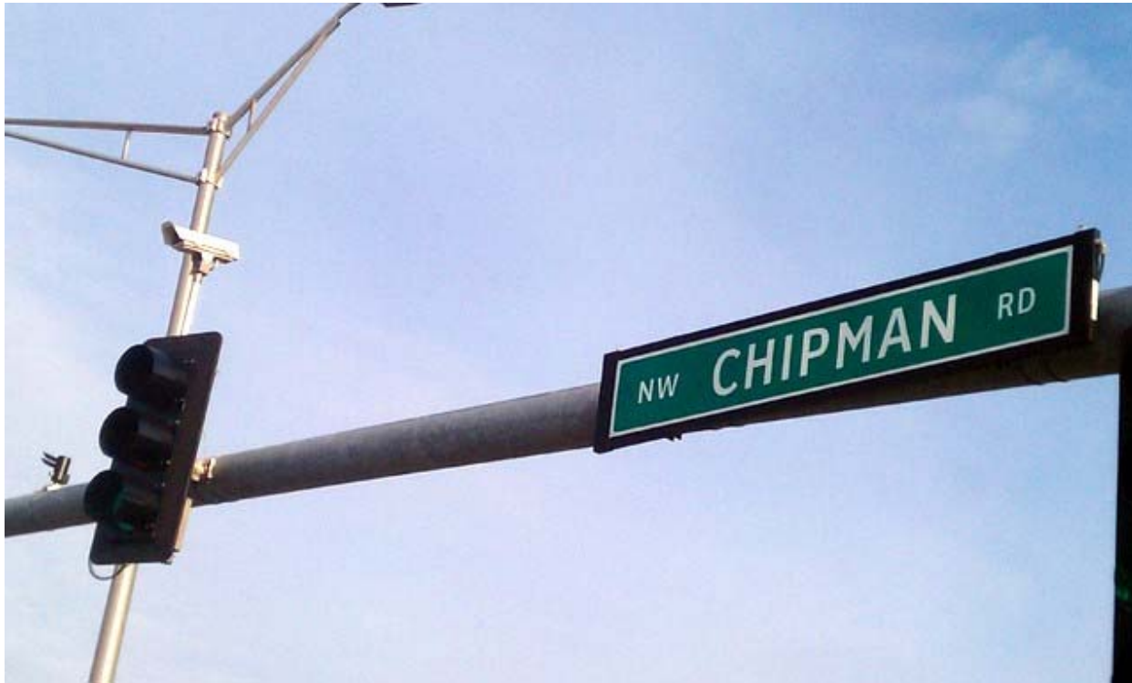
A mast arm on Chipman Rd. with mounted Internet Protocol video camera for vehicle detection.
