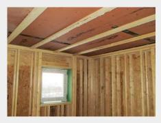
Inner and outer wall framing is typically framed with 2×4s at 16" o.c. Inner and outer wall studs do NOT need to be offset. The distance between inner and outer wall framing varies depending on desired R-value. Overall depth typically does not exceed 16" (refer to insulation manufacturer's installation guidelines.)
