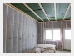
Dense-blown cellulose, blown fiberglass, or open-cell spray foam can be installed to full depth. If using a combination of products, proper attention must be paid to the ratio of air-impermeable insulation (closed-cell foam) to air-permeable insulation (fiberglass, cellulose) or condensation problems could occur.
