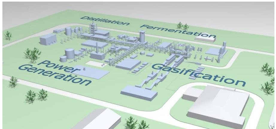
cooled and cleaned before being fed to naturally occurring bacteria. These patented bacteria convert the synthesis gas into ethanol, which is purified for use as fuel in the transportation market.
