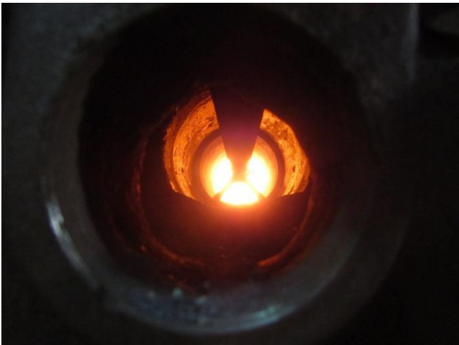
RTP Green Fuel Flame
