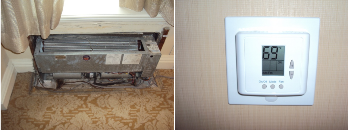
Figure 16. Photograph of an Island Air PTHP unit and a WiSuite OBC thermostat at the Mayflower Renaissance.
