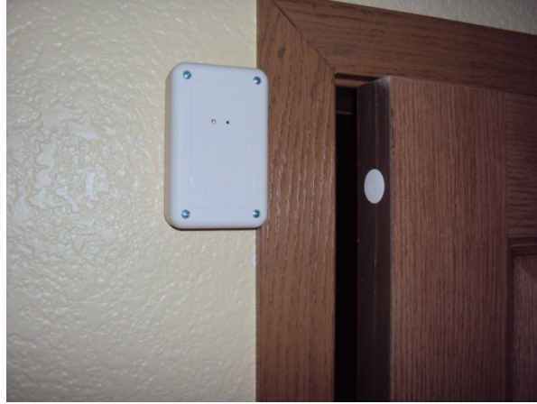
Figure 14. Photograph of a Onity Wireless Door Switch at TownePlace Suites Los Angeles LAX/Manhattan Beach.
