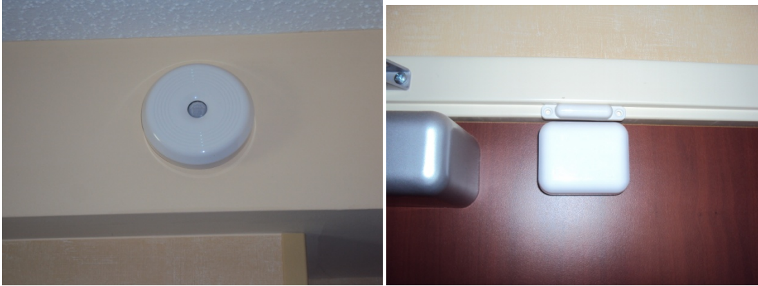
Figure 20. Photograph of a Schneider Electric Wireless Occupancy Sensor and Wireless Door Switch
