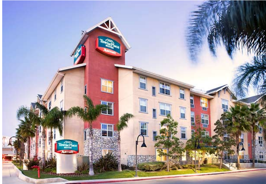
Figure 12. Photograph of the TownePlace Suites Los Angeles LAX/Manhattan Beach.
