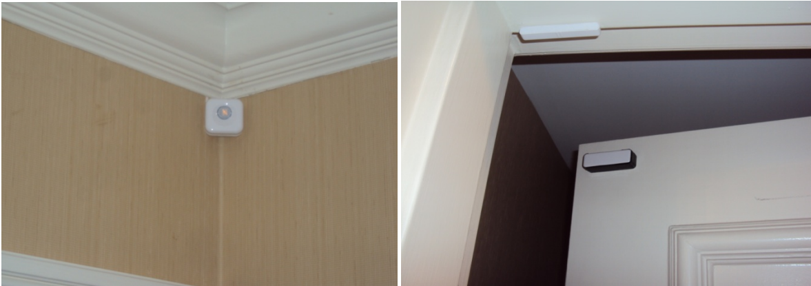
Figure 17. Photograph of a WiSuite Wireless Occupancy Sensor and a Wireless Door Switch at the Mayflower Renaissance.
