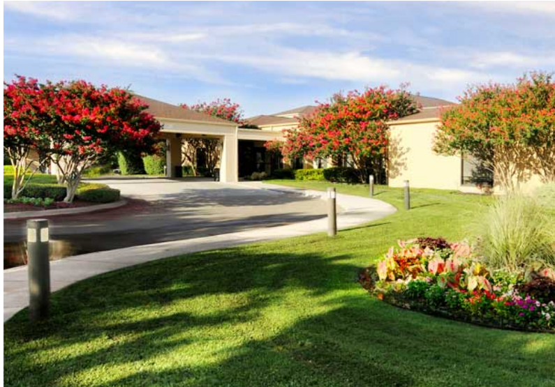
Figure 4. Photograph of the Courtyard Dallas Addison/Midway.
