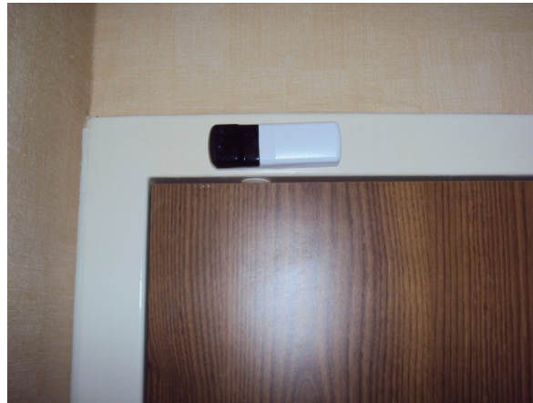
Figure 9. Photograph of an Inncom Wireless Door Switch at the Courtyard Dallas Richardson at Spring Valley.
