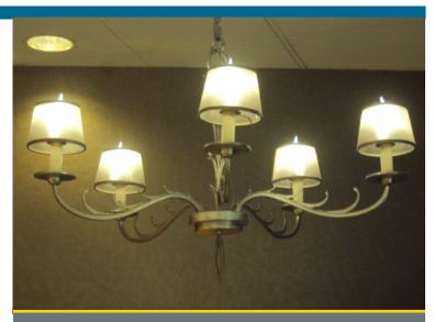
Fixtures using light-emitting diodes are becoming cost effective for interior use. Lobby chandeliers were retrofitted to replace incandescent lamps with light-emitting diodes. The hotel already used compact fluorescent lamps in most other fixtures.
