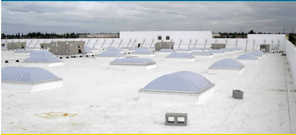
(Left) At The Home Depot store in Lodi, California, increasing the number of skylights to improve daylighting and customer experience was determined to be cost effective. Skylights from the Lodi store are shown at roof top level. (Right) In The Home Depot store, the checkout area is the focus of many of the skylights. Daylighting sensors adjust the lighting level from 100% to 50% or 0%. In this photo, the 0% lighting level is active, where the overhead lights in the upper left are completely off.
