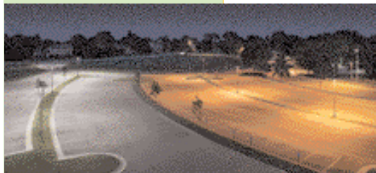
The parking lot lighting demonstration comparing LED (left) and high-pressure sodium (right) shows the even light distribution and good color rendering of LED lighting.
