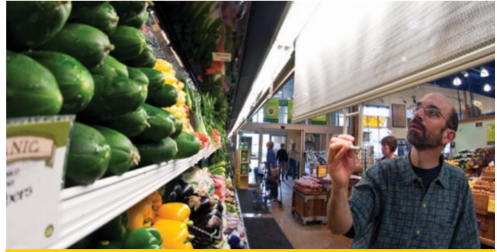
Whole Foods Market selected efficient lighting and night curtains for open produce cases.
