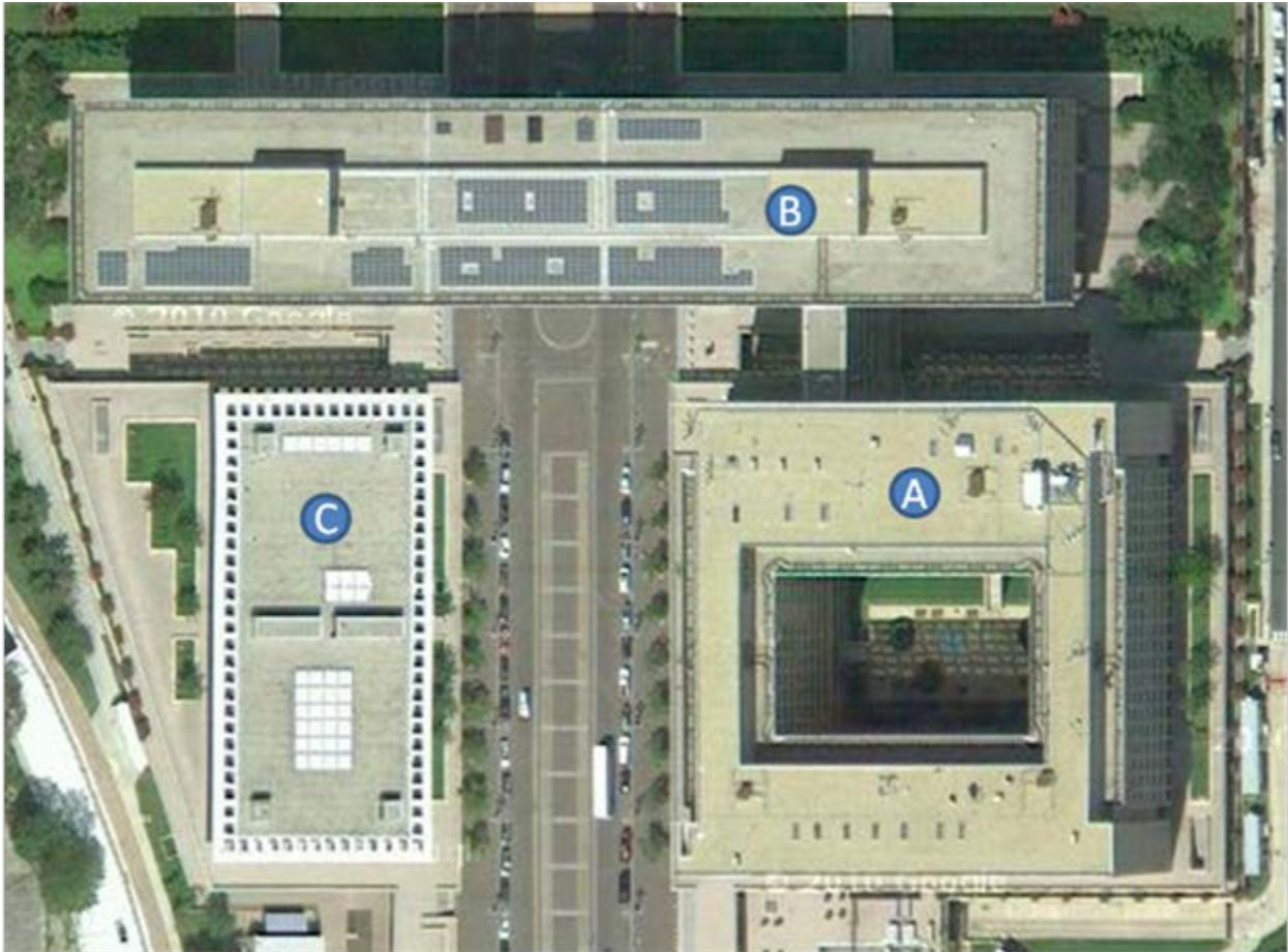
Figure 2. Aerial view of the Forrestal Building showing the South Building (A), the North Building (B) and the West Building (C).
