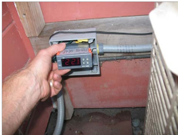
Figure 2-3. Fan controller and outdoor temperature sensor
