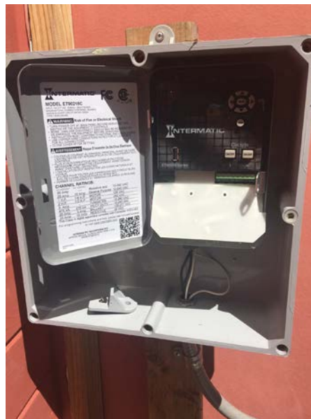
Figure 2-9. Whole-house exhaust fan timer deployed for OTSVC field testing
