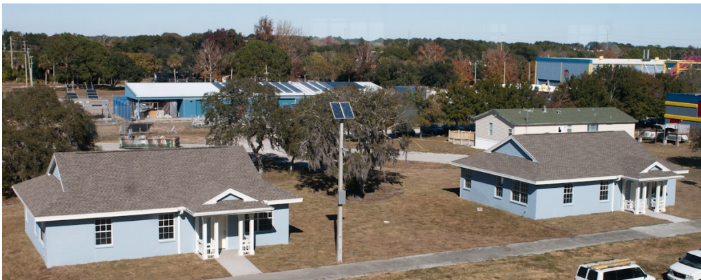
Figure 3-4. Flexible residential test structures on FSEC campus
