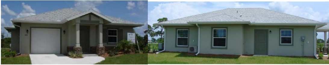
Figure 3-24. South Sarasota Habitat for Humanity test house, front and side views
