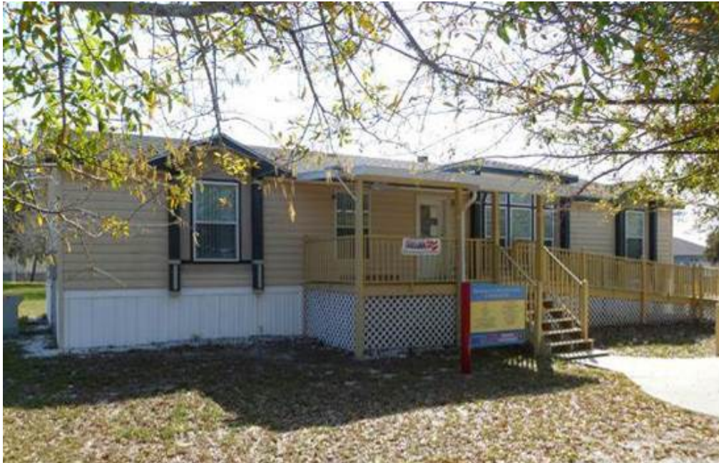
Figure 2-1. Florida Solar Energy Center manufactured house laboratory. The north side is shown.
