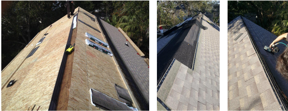
Figure 42. Panel and roofing during installation
