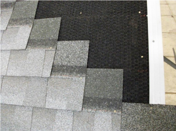
Figure 12. Installation of shingles and ridge vent
