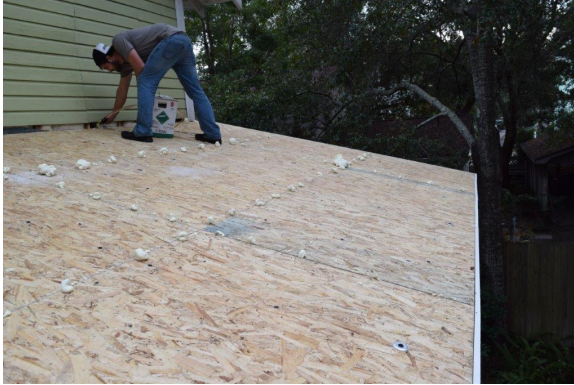
Figure 33. Retrofit panels sealed at panel-to-panel edges
