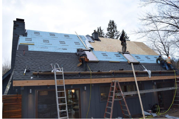
Figure 47. Roofing the back of the main roof
