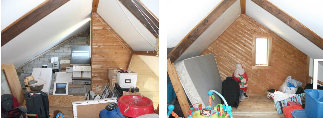
Figure 19. Michigan addition roof (Rafters shown are decorative.)
