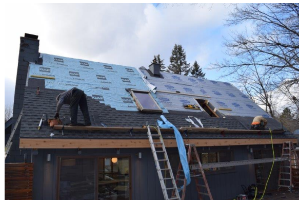
Figure 46. Skylights were removed and reinstalled after panels
