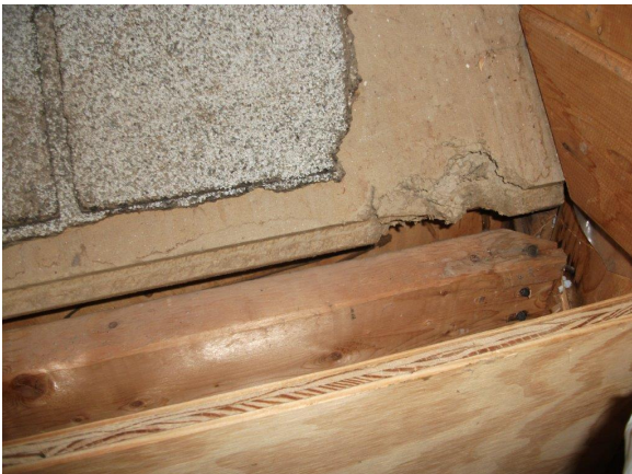
Figure 8. Michigan main house existing fiberboard roof deck/ceiling
