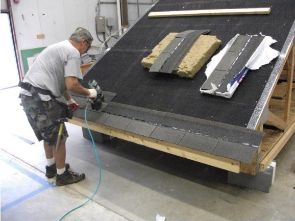
Figure 11. Installation of shingles
