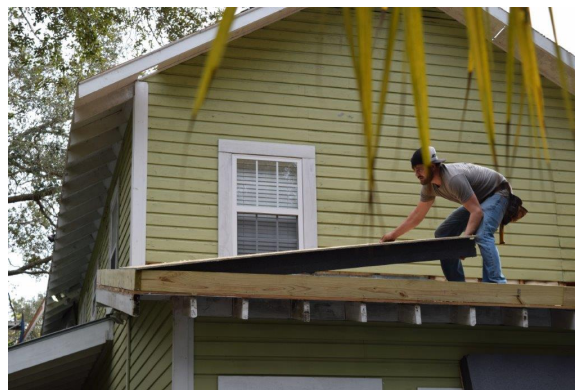
Figure 30. The first retrofit panel was placed on the one-story roof
