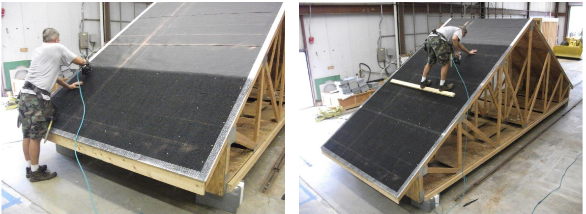
Figure 10. Installation of ventilation mat
