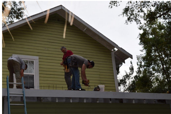
Figure 32. Panels were screwed into rafters
