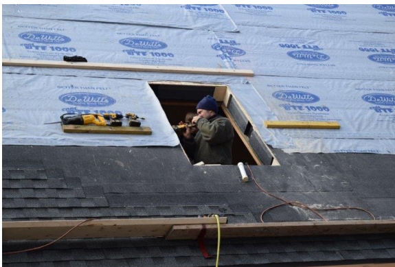
Figure 46. Skylights were removed and reinstalled after panels
