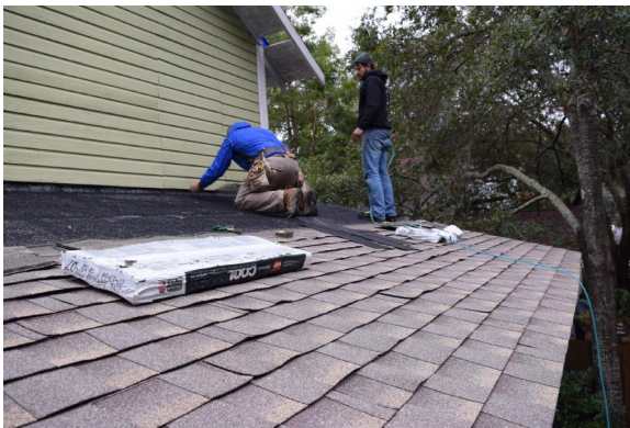
Figure 35. Ventilation mat and shingles on one-story roof
