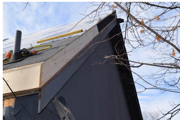
Figure 45. Nailing curbs installed after the retrofit panels
