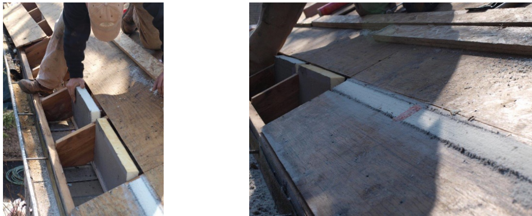
Figure 23. Example eave insulation method
