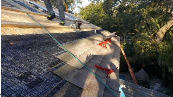
Figure 41. Ventilation mat and shingle installation
