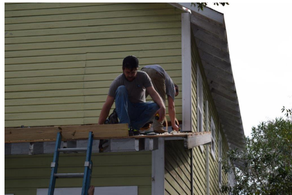
Figure 29. A 2x8 “curb” was installed before the retrofit panels
