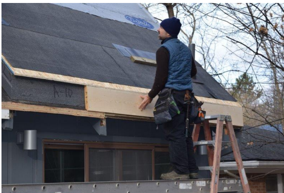
Figure 45. Nailing curbs installed after the retrofit panels
