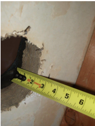
Figure 8. Michigan main house existing fiberboard roof deck/ceiling
