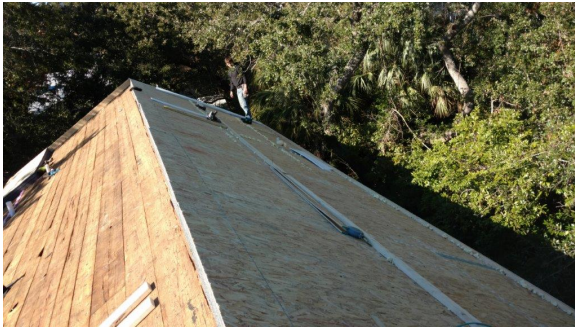
Figure 40. Panel installation progress on the second-story roof
