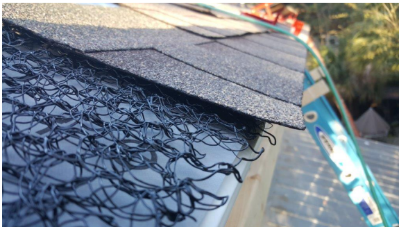
Figure 41. Ventilation mat and shingle installation
