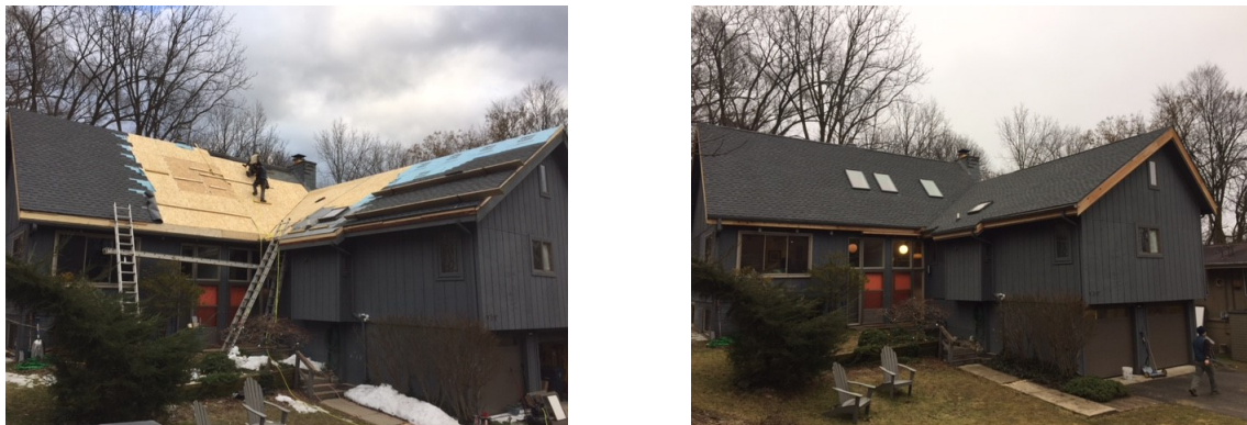
Figure 49. Installation progress and installation complete
