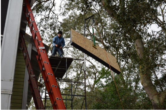
Figure 39. Panels were hoisted manually to the second-floor roof
