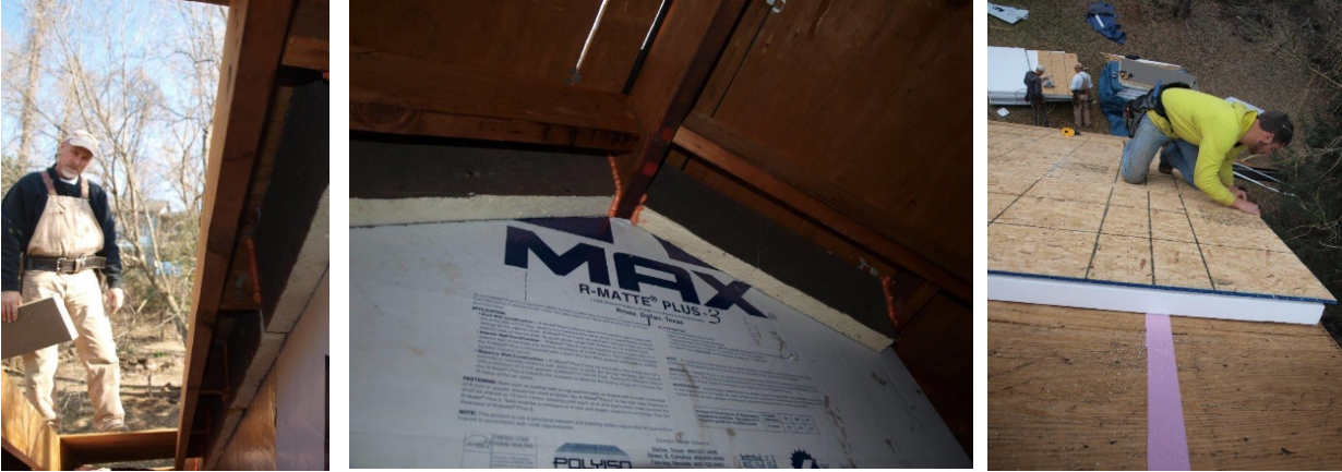
Figure 24. Example gable wall insulation method
