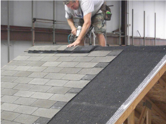
Figure 12. Installation of shingles and ridge vent
