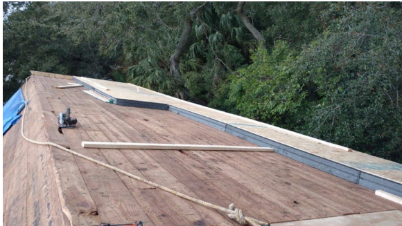
Figure 40. Panel installation progress on the second-story roof
