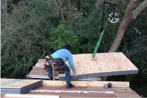
Figure 39. Panels were hoisted manually to the second-floor roof
