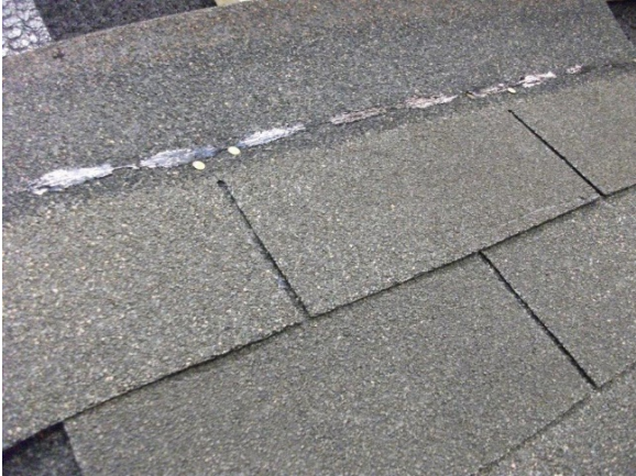
Figure 11. Installation of shingles
