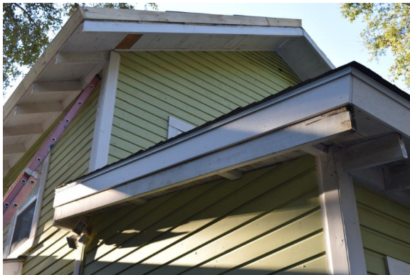
Figure 36. First-story roof complete
