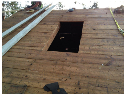
Figure 25. Construction access to attic at roof deck
