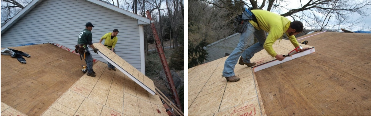
Figure 2. Example installation of retrofit panels during a reroofing effort
