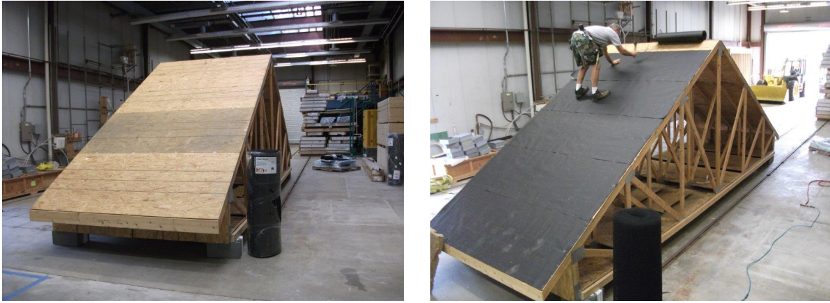
Figure 9. Mock-up roof deck assembly and installation of underlayment
