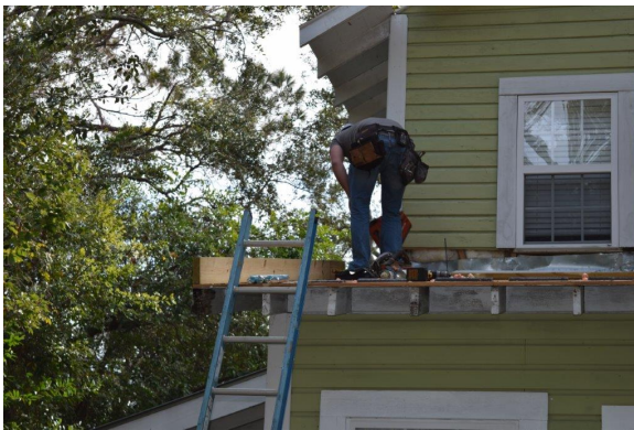
Figure 29. A 2x8 “curb” was installed before the retrofit panels
