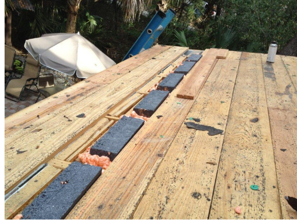
Figure 28. Rigid foam insulation at eaves
