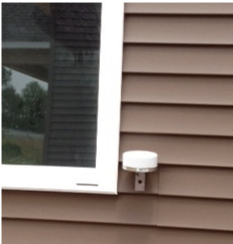
Figure 7. Exterior sensor attached to the cladding
