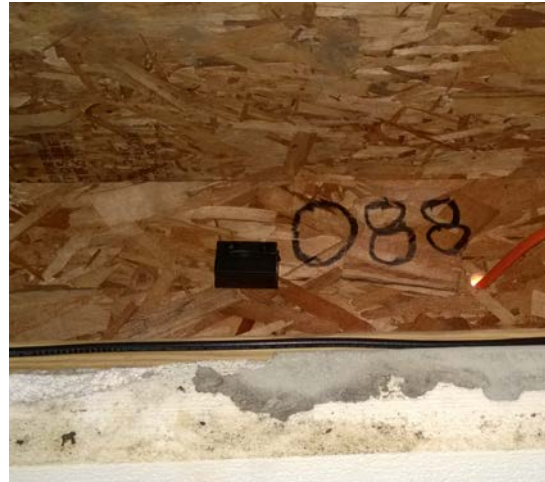
Figure 6. Sensor installed in the rim joist
