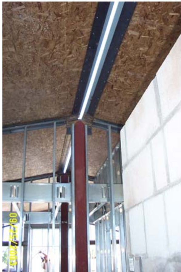
Figure 31. Structural insulated panels provide the air and thermal barrier for the roof
