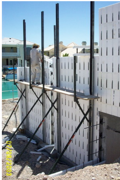
Figure 29. Insulated concrete forms make up the exterior shell of the home.
