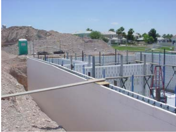
Figure 30. Insulated concrete forms were used to form the walls of the basement
