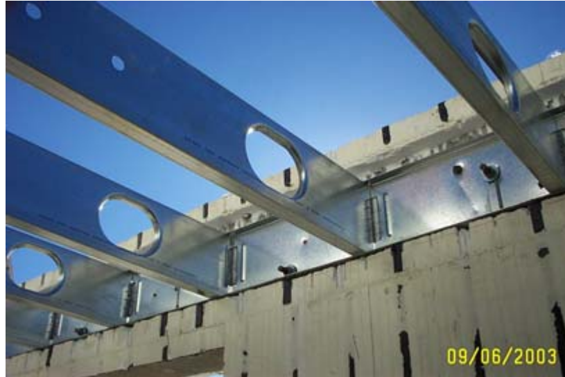
Figure 28. Steel beams were used for structural framing and are anchored into the insulated concrete form wall.
