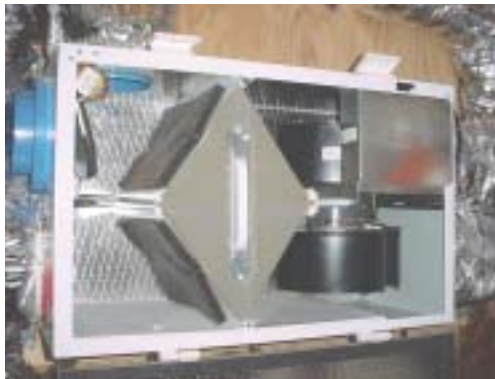
Energy recovery ventilator tempers fresh outdoor air before delivering to HVAC equipment
