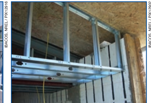
Insulated concrete forms, steel beams, and structural insulated panels make up the building enclosure.
