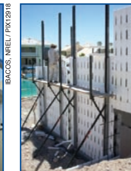
Steel beams (left) for structural framing are anchored into the insulated concrete form wall, and (right) insulated concrete forms make up the exterior shell of the home.
