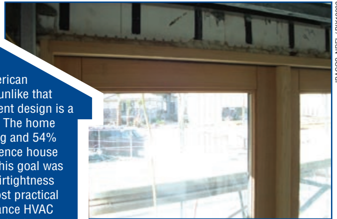
Expanding foam insulation seals the windows to prevent air infiltration.
