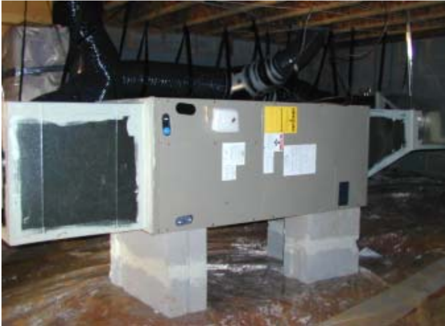
Figure 7. Locating mechanical equipment responsible for air movement in a conditioned space, such as this conditioned crawlspace, means that it is not subject to the cold and extreme hot and humid circumstances that it would experience if it was located in an attic, vented crawlspace, or the outdoors.
