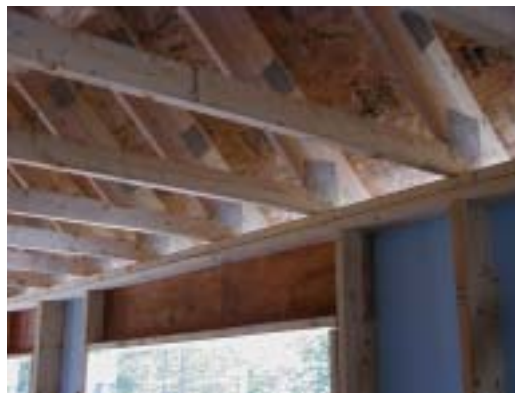
Figure 13. Energy trusses, also known as a “slider truss”
