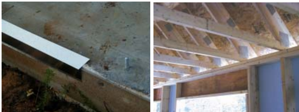
Figure 49. Flashing (left) and slider trusses (right)
