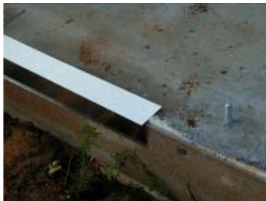
Figure 61. Flashing with FiberCement board
