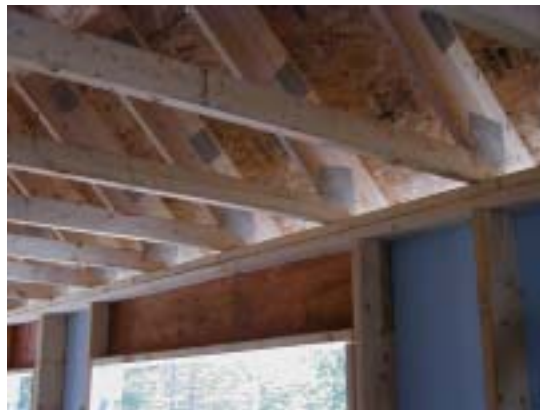
Figure 69. Slider truss
