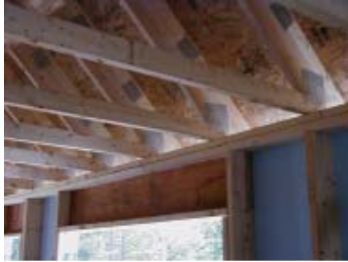
Figure 55. Slider truss
