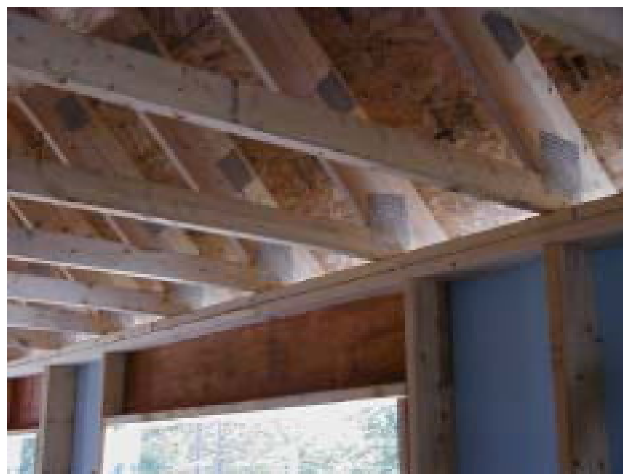
Figure 35. A “slider” truss
