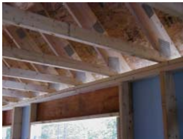
Figure 42. Slider truss
