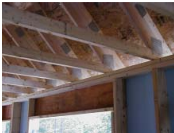
Figure 19. Energy truss, also known as a “slider truss”
