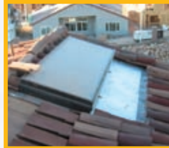
Solar hot water heater on the roof uses the desert sun to heat water for the home.
