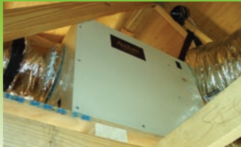
Dehumidifier/ventilator system filters outdoor air before it is distributed.
