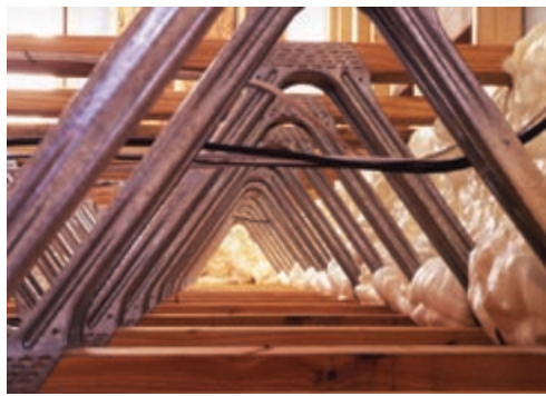
Open web trusses provide space within the building enclosure to run electrical wires and ducts.
