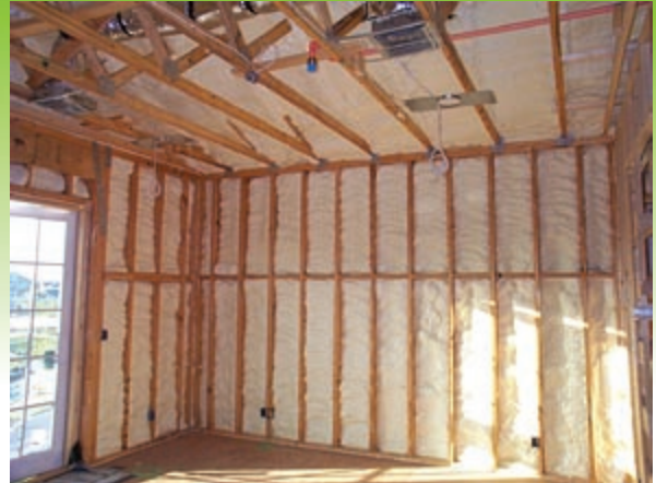
The second floor is insulated with spray foam, minimum R-19.
