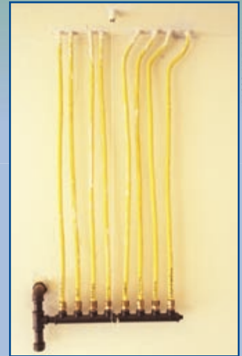
This manifold piping distribution system is easier to install than traditional systems.
