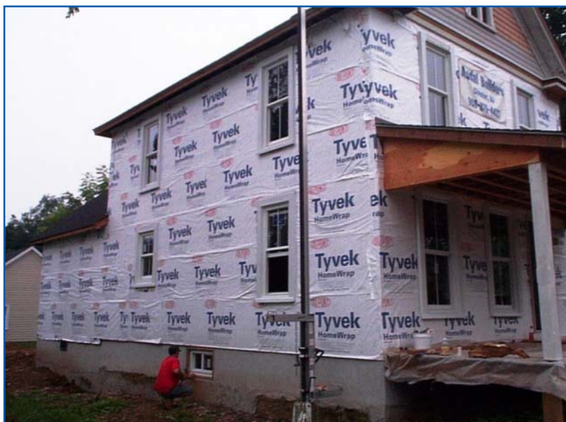
Air barrier on outside of house
