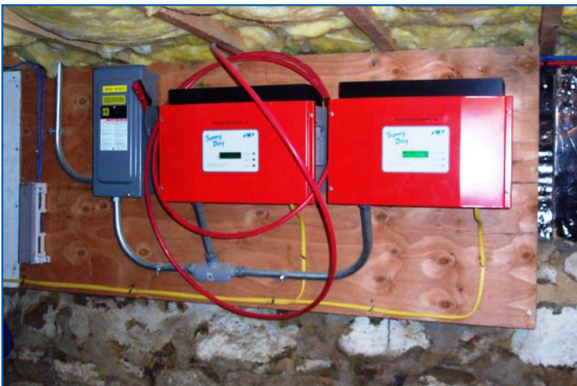
PV system inverters
