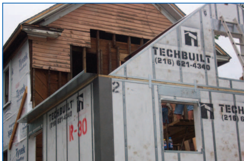
Addition construction using foam panels
