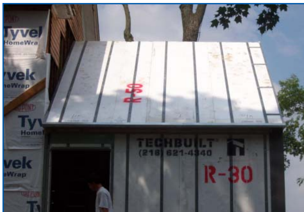
R-50 roof and R-30 wall panels
