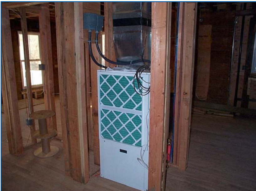
Ground source heat pump in conditioned space
