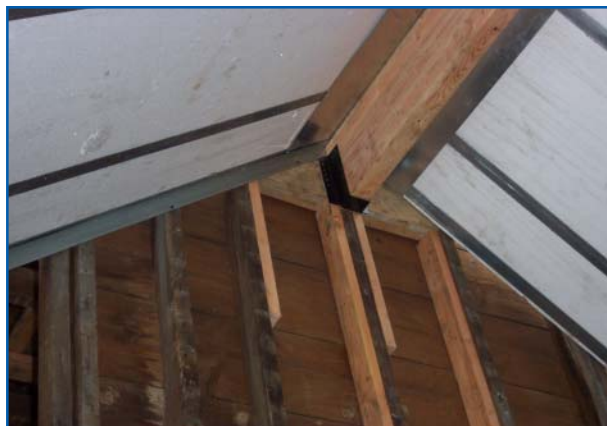
Ridge beam for roof support
