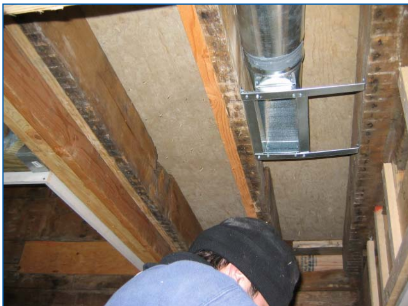
All duct joints sealed
