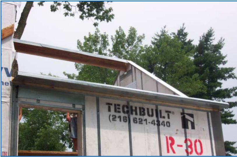
Ridge and eave supports for roof panels
