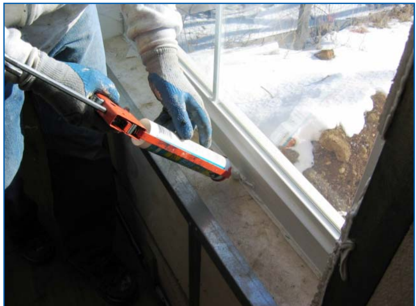
Air sealing around windows
