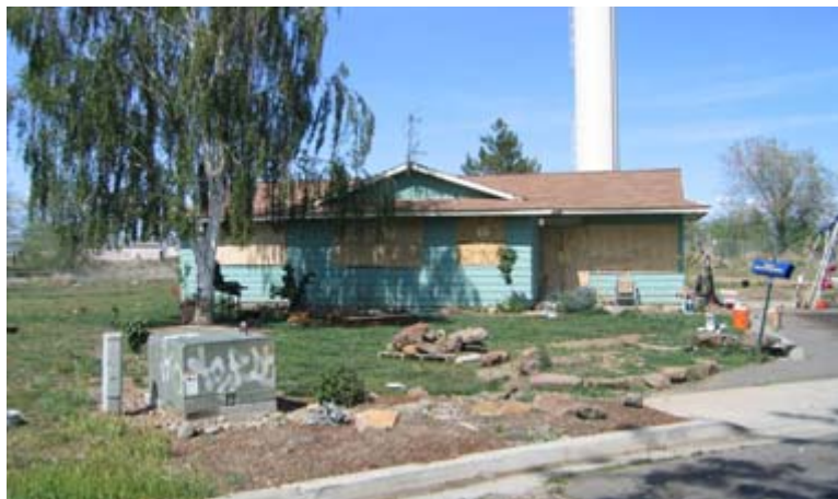
Figure 1. One of the boarded-up homes at Adam's View scheduled for rehabilitation
