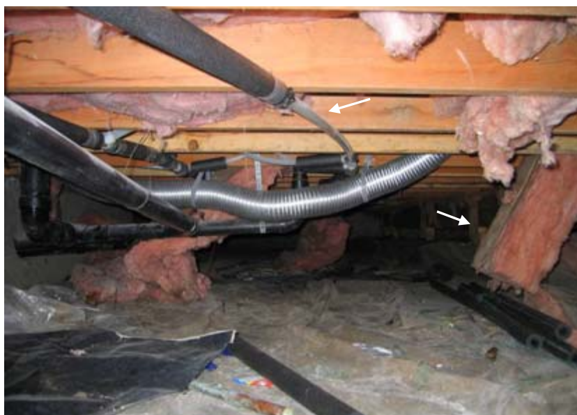
Figure 14. Crawlspace of Unit #303
