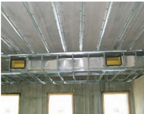
Well-sealed, fiberglass ductboard is completely enclosed in conditioned space.
