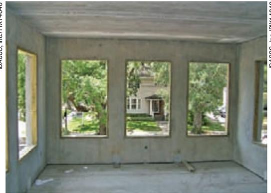
Openings for windows and any other penetrations required careful design and placement in the pre-cast concrete system.
