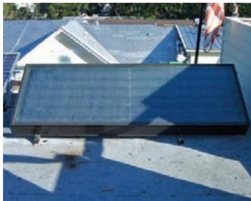
A solar thermal hot water system preheats incoming water.
