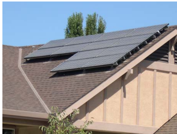
Figure 35. PV system-mounted above roof surface to dissipate heat
