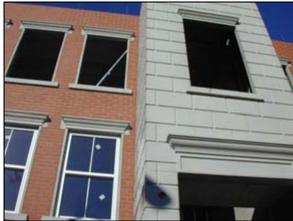
Figure 30. Crown lintels over windows
