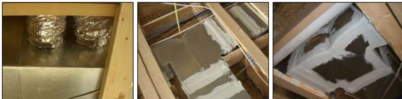
Figure 43. Using pressure-sensitive aluminum foil tape and mastic to seal intersections of ducts
