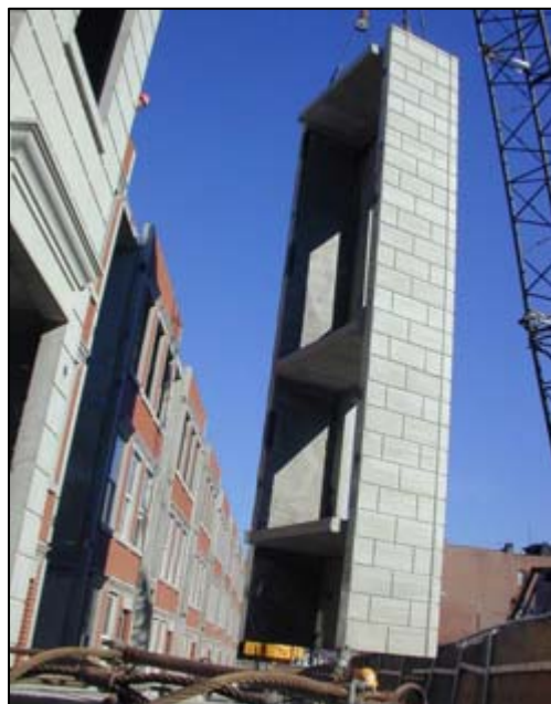
Figure 31. Precast concrete panelized wall system
