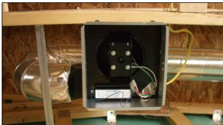
Figure 44. Improperly installed ventilation fan
