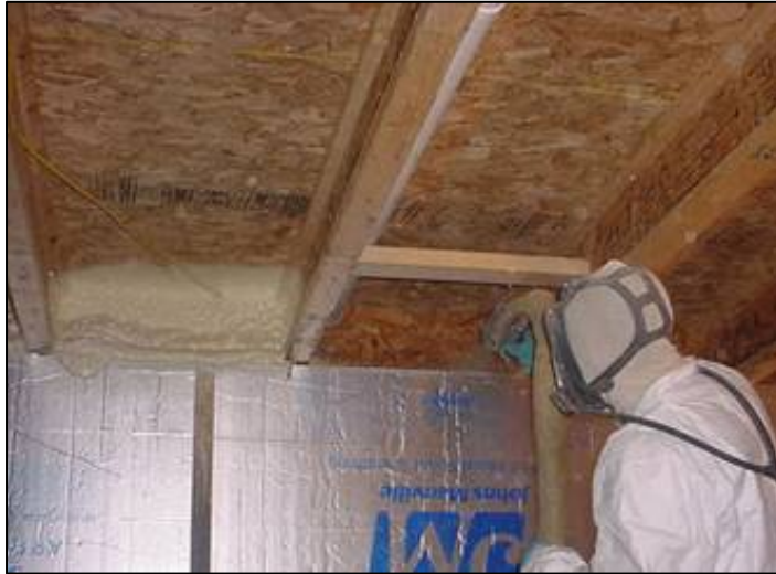
Figure 42. Insulating the box sills of all floors
