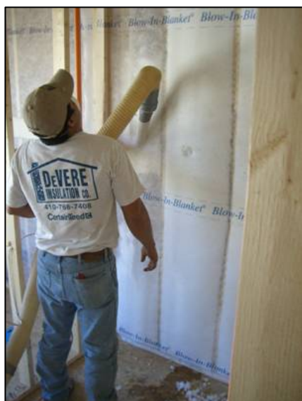
Figure 40. Blanket insulation
