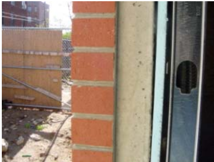
Figure 32. Extruded polystyrene board between the exterior walls and interior metal studs
