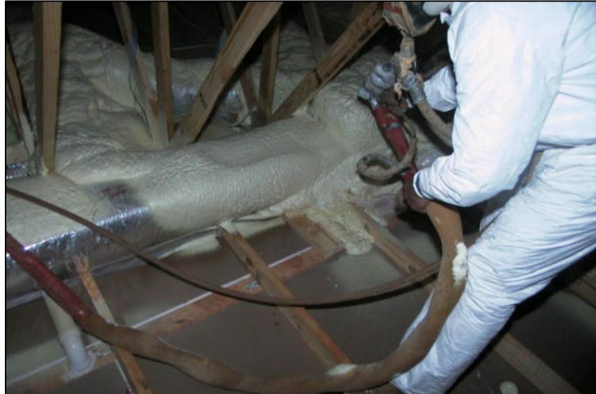
Figure 52. Insulating ducts with closed-cell polyurethane foam
