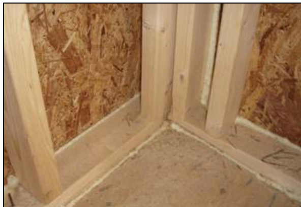
Figure 39. Low-expansion foam used to air seal stud cavities
