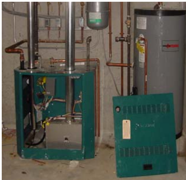
Figure 33. Sealed-combustion, direct-vent, gas-burning Burnham Revolution boiler with a 65-gal. Bradford-White automatic-storage water heater
