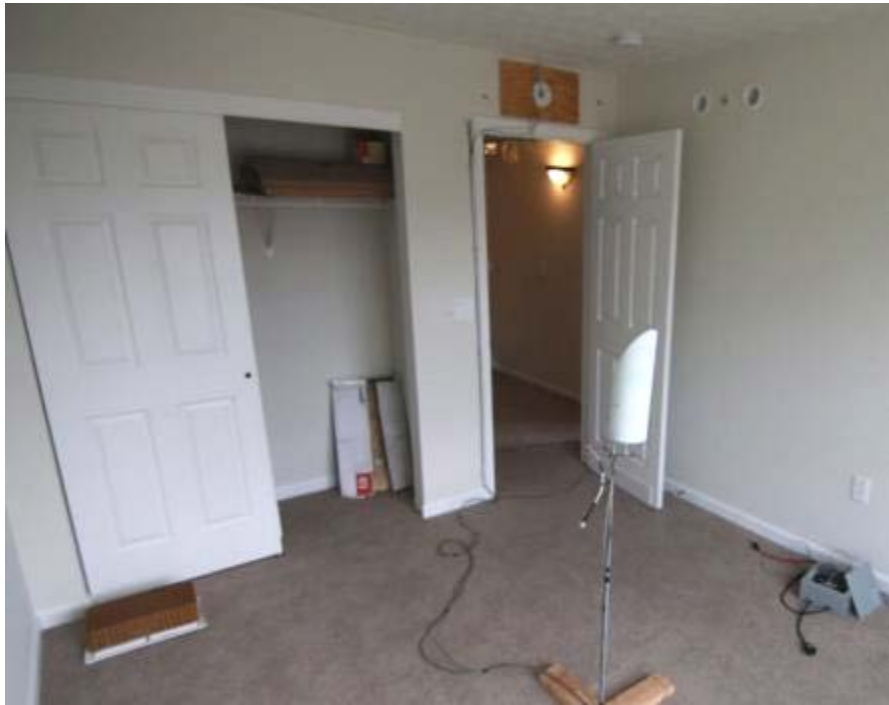
Figure 3. Photograph from the interior of bedroom 3 showing the supply outlet and air temperature measurement stand
