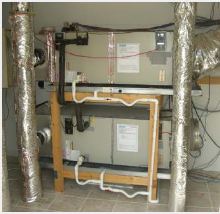
Figure 1. AHUs for SEER 13 (top) and SEER 22 (bottom) 2-ton heat pumps can be connected to indoor or attic ducts.
