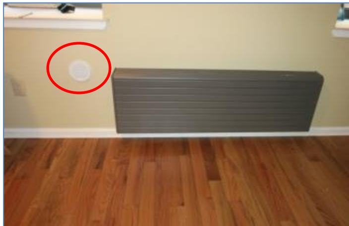
Figure 4. Incorrect airlet installation
