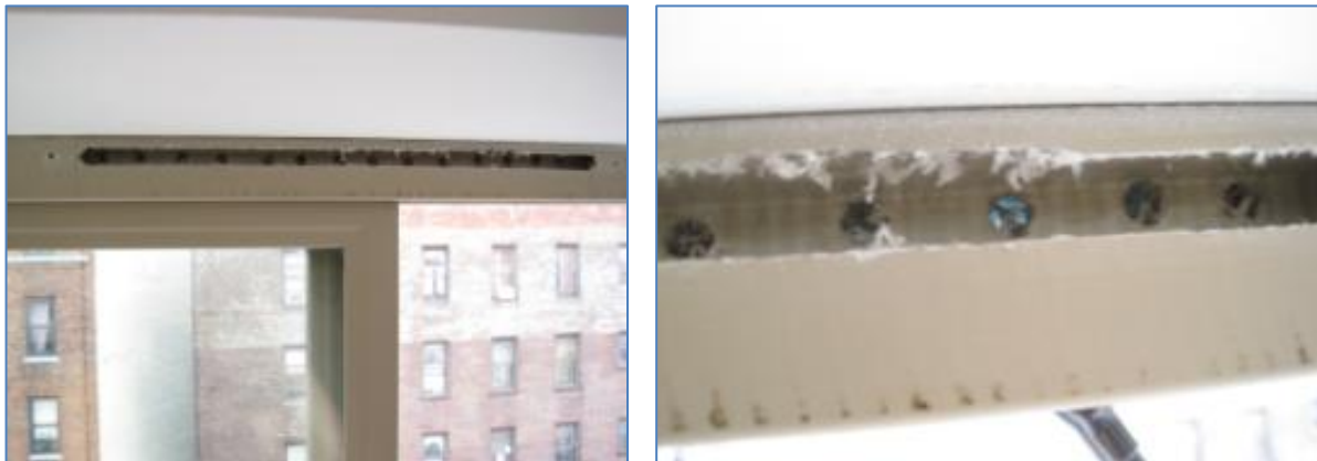
Figure 3. Cut for trickle vent in window frame (left). Close-up of opening (right)
