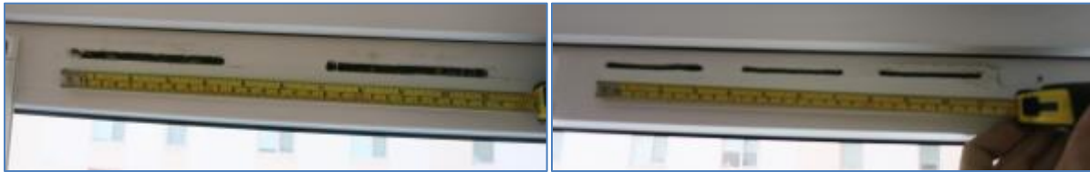
Figure 2. Examples of inconsistent trickle vent installation
