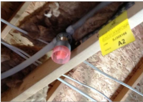
Sprinkler rough install
