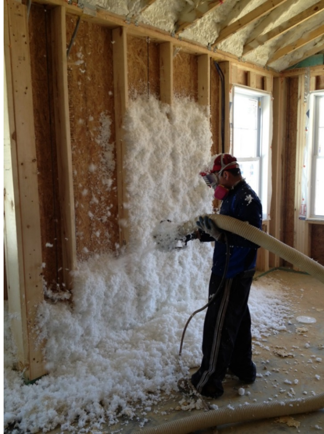
Figure 18. Installation of Johns Manville Spider insulation
