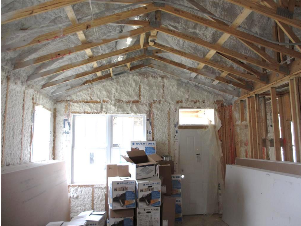
Figure 19. Spray-applied Spider insulation
