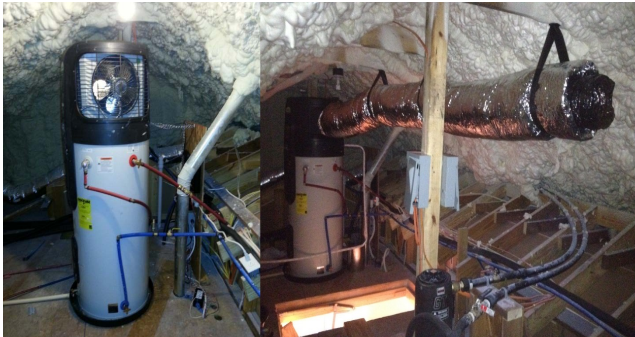
Figure 27. Savannah Gardens Lot 207 HPWH in the encapsulated attic before the exhaust duct was installed (left) and after the exhaust duct was installed (right)
