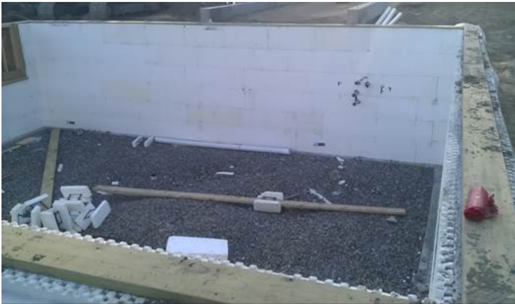
Figure 2. The ICF foundation in Lincolnville. Image from Black Bros. Builders
