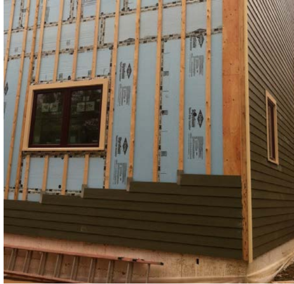
Figure 8. Fiber cement clapboard siding installed on furring strips
