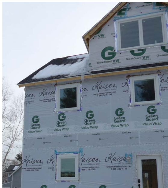
Figure 6. A later BrightBuilt Home in which house wrap was installed outside of the foam insulation
