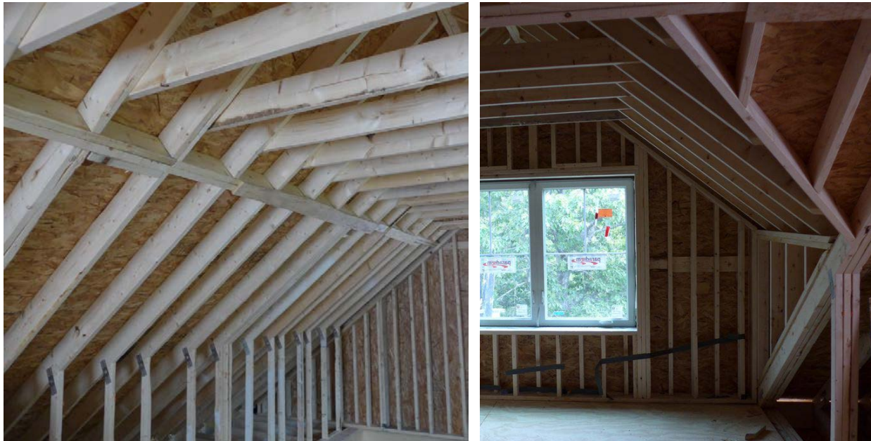
Figure 9. The tilt-up roof (left) and factory-assembled dormer (right)
