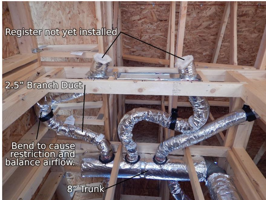
**Figure 8. Small-diameter trunk-and-branch plenum on the third floor of Home A1**
