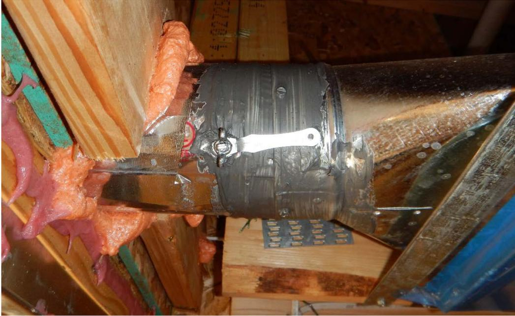
**Figure 10. Register for the builder’s standard system, showing a balancing damper and mastic**
