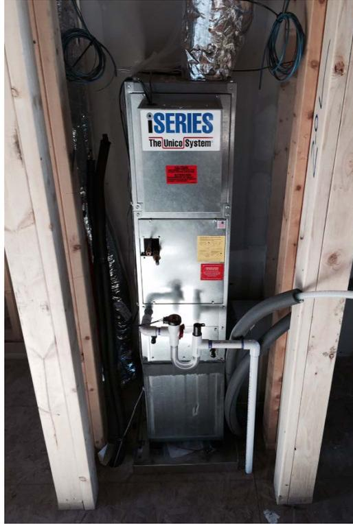
**Figure 9. Small-diameter upflow air handling unit on the second floor of Home A2**
