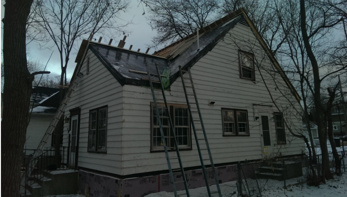
Figure 16. The air/water membrane applied to the existing roof deck
