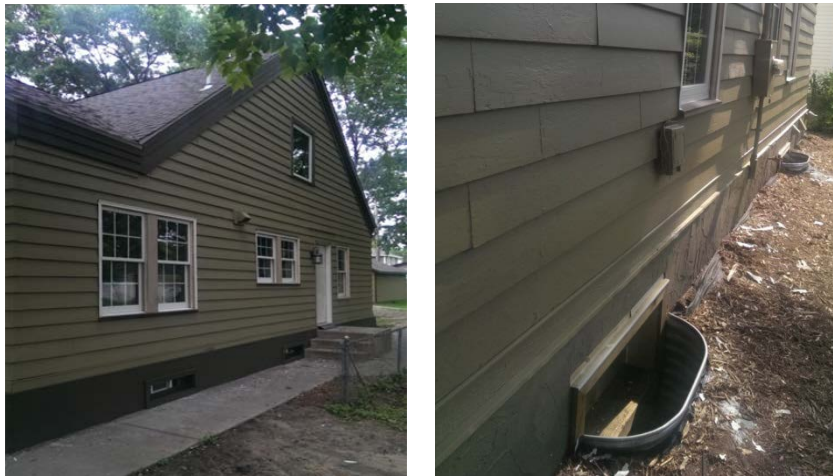
Figure 12. Completed foundation insulation with trim and windows
