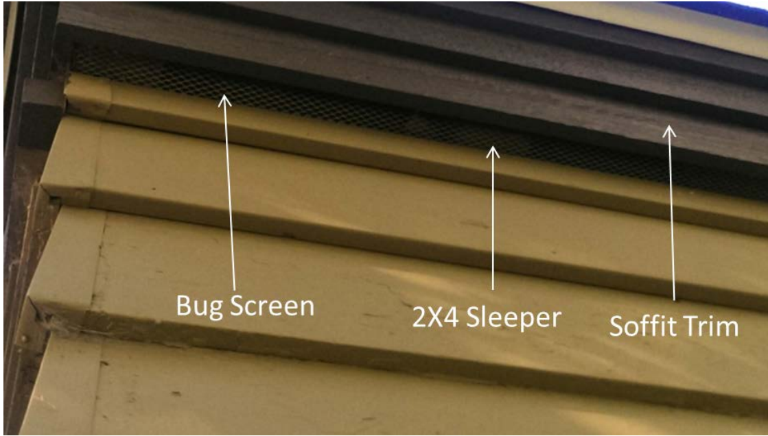
Figure 20. Trim boards attached to the vertical sleepers form air intake channels to the ridge
