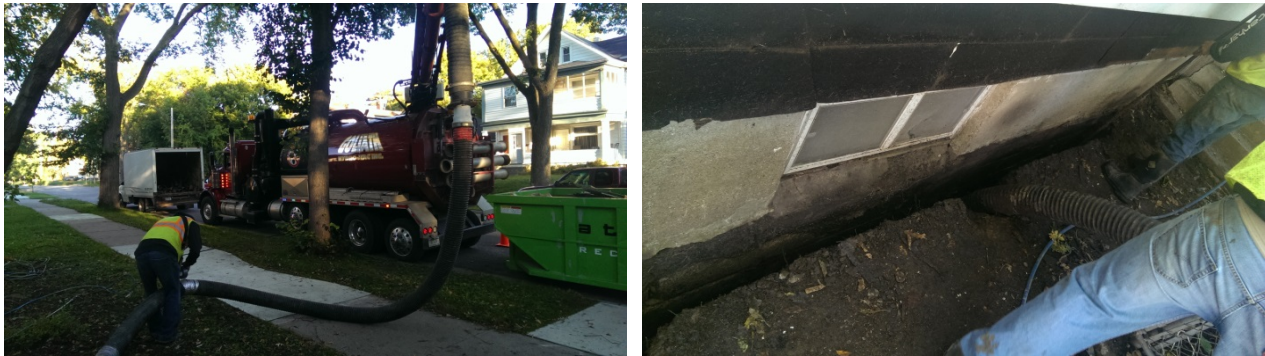
Figure 2. Hydro-vac truck and high pressure water nozzle cutting a narrow trench
