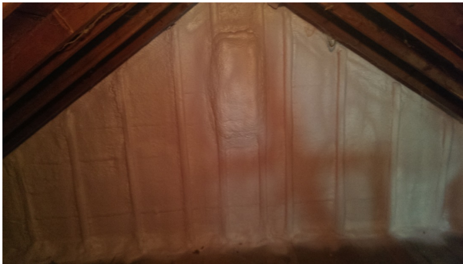
Figure 15. Interior-applied foam on the gable end
