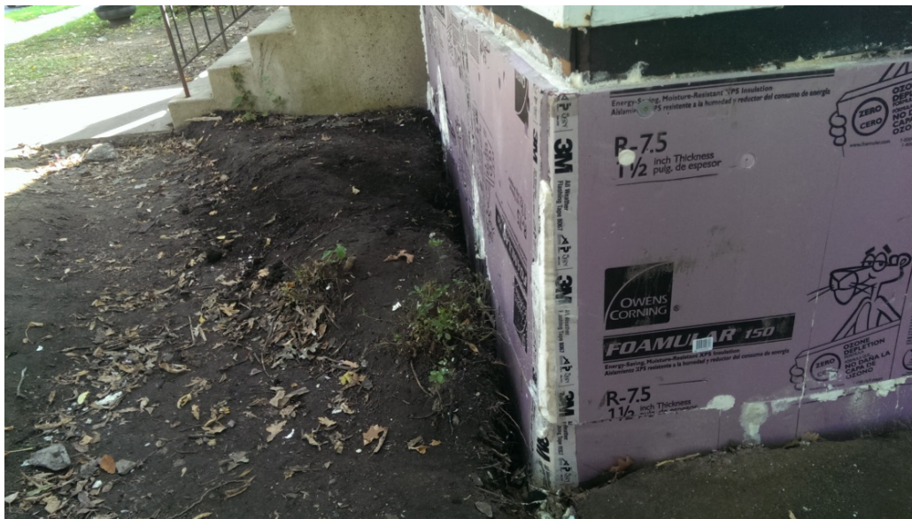
Figure 10. Smooth, flat surface created by the rigid insulation
