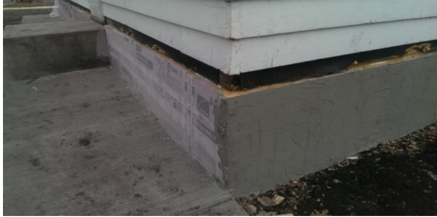
Figure 11. Foam system with stucco applied to one side
