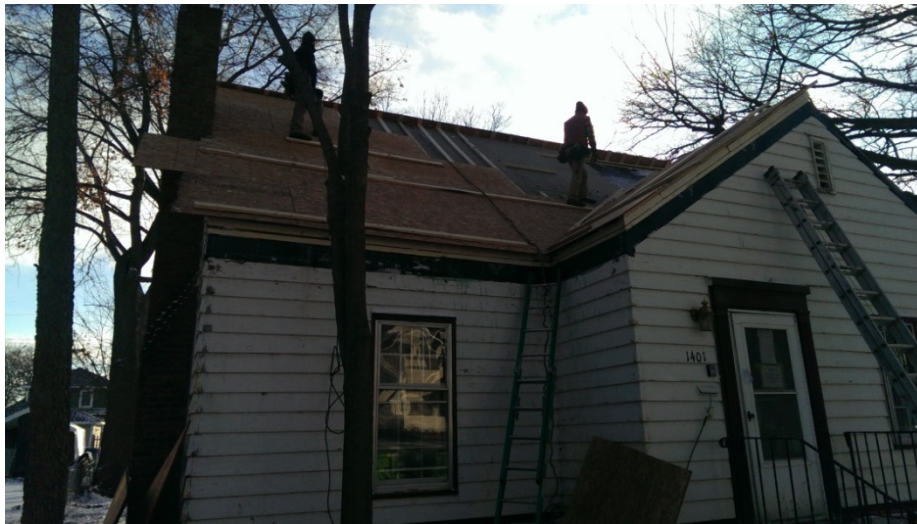
Figure 17. Installation of the insulation, furring strips, and new roof deck
