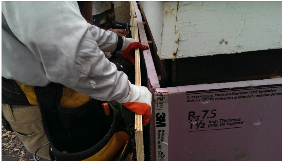
Figure 9. Above-grade rigid XPS foam held flat with attached plywood
