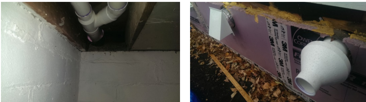
Figure 14. Exhaust system sleeve installed prior to application of exterior insulation
