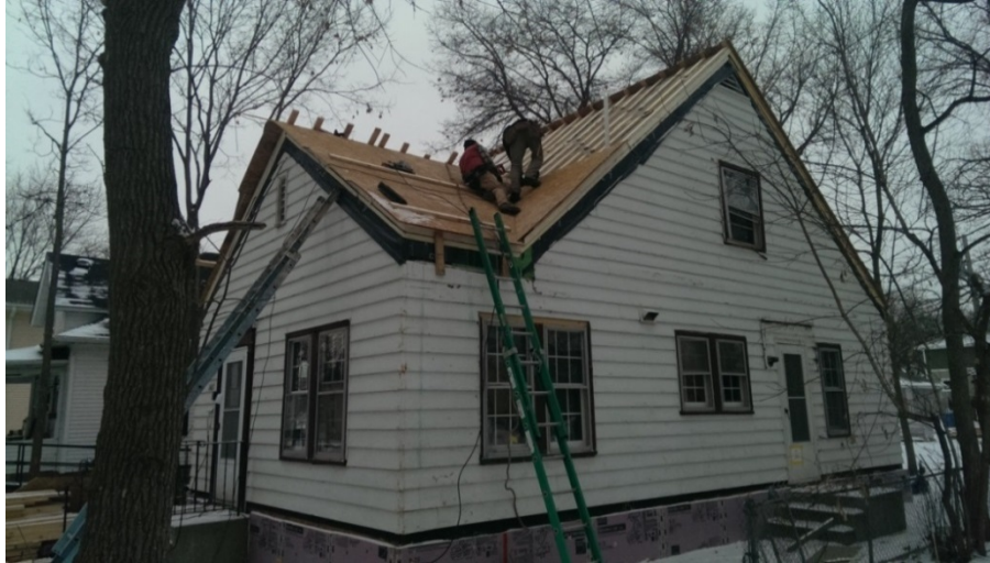
Figure 18. Furring strips and roof sheathing forming an air channel for ventilation
