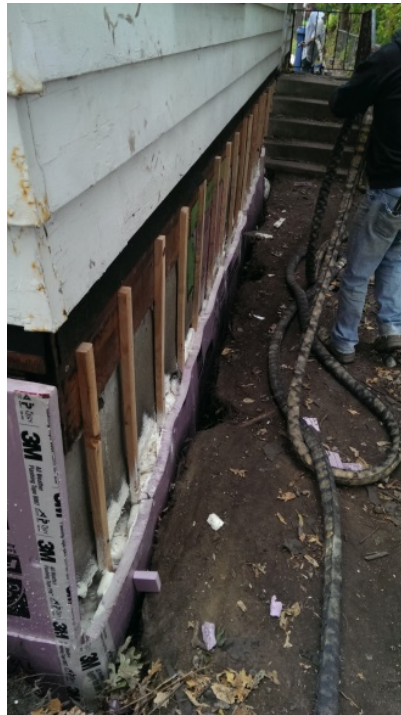
Figure 8. Pouring the liquid foam into the 1-in. cavity
