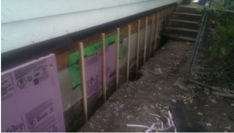
Figure 7. Furring strips to hold the above-grade rigid form 1 in. from the foundation
