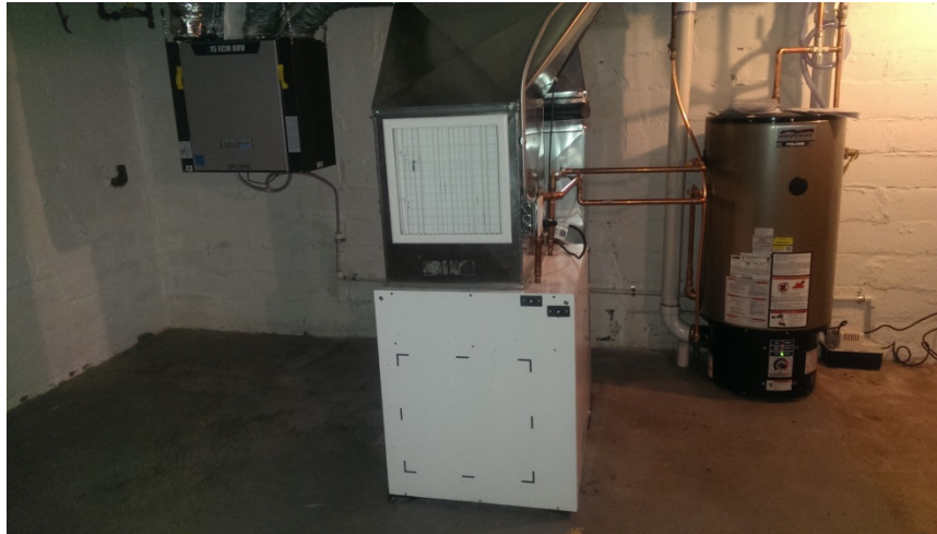
Figure 13. Combi system installed in the project house, including an HRV
