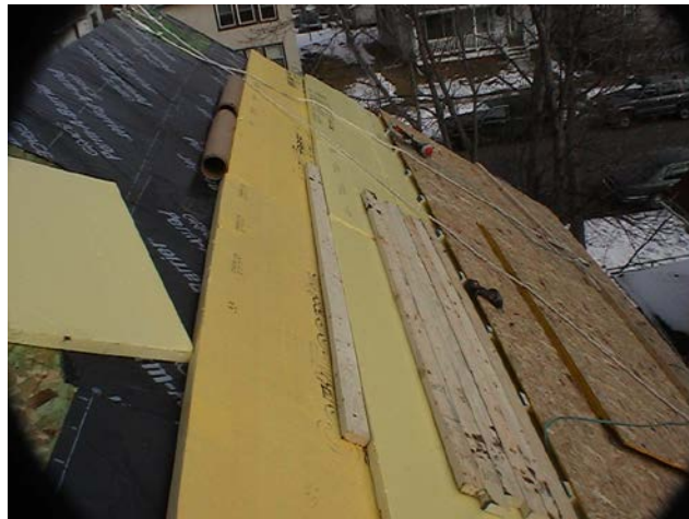
Figure 4. Details for roof overcoat applied to a 1-½-story home
