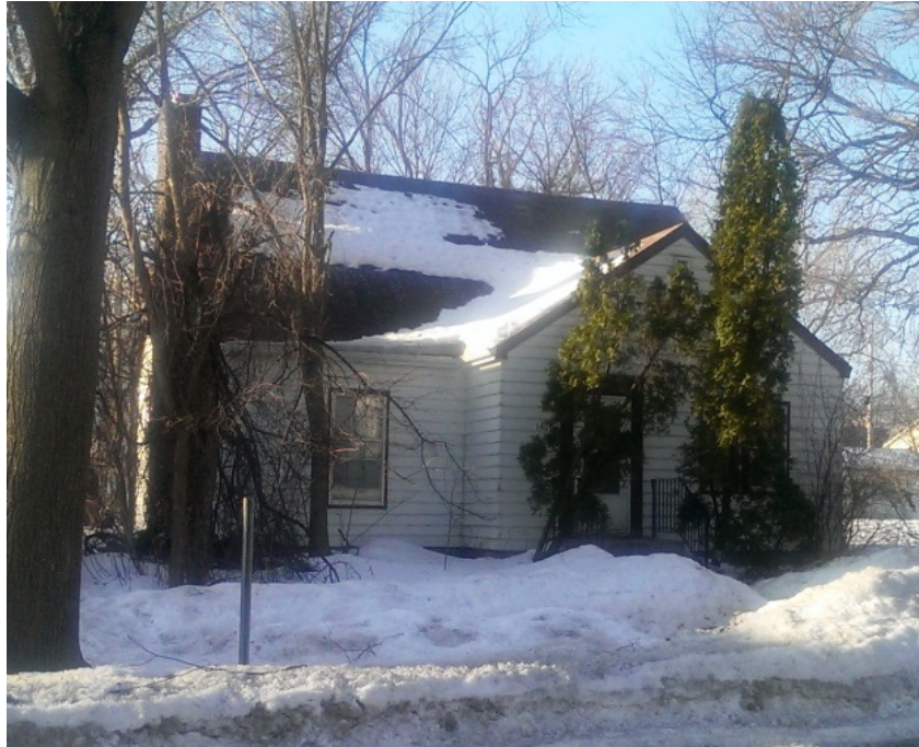
Figure 1. Demonstration home in Minneapolis, Minnesota
