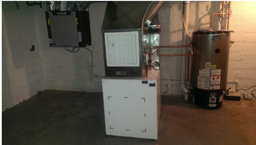
Figure 5. Example of the combi space and water heating system
