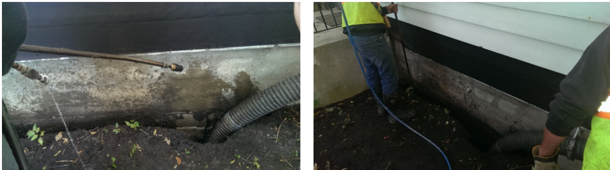
Figure 6. The hydro-vac high-pressure water wand and vacuum used to create the trench
