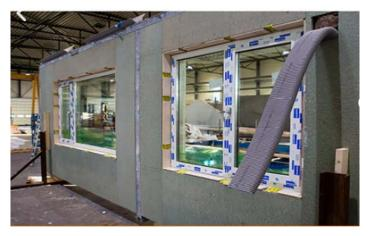
Figure 10. Ducting integrated into Renolution facade panel
