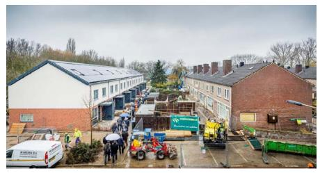
Figure 2. Typical row house typology in the Netherlands before (right side) and after (left side) retrofit Photo courtesy of Energiesprong
