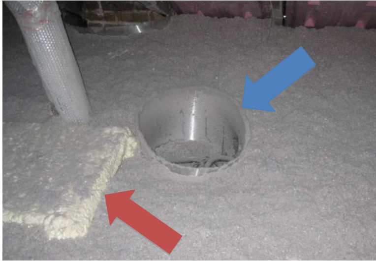
Figure 10. Bath fan housing cover encased in foam sealant (red arrow) and electrical junction box surrounded by metal insulation dam (blue arrow)
