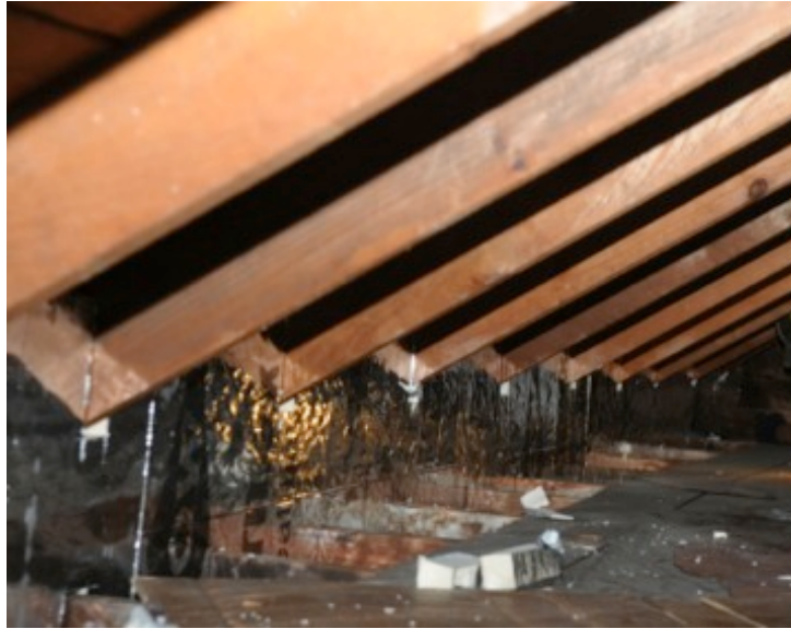
Figure 19. Foil-faced polyisocyanurate insulation notched around roof and ceiling framing (Photo credit: E. Haber, printed with permission)
