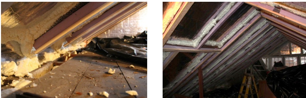
Figure 25. Left: Extruded polystyrene and wood furring strip used to extend rafter cavity; Right: Attic with rafter cavities extended in preparation for mineral fiber insulation (Photo credit: S. Marchese, printed with permission)
