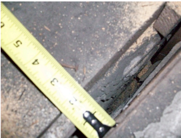
Figure 2. Furring cavity between brick masonry and interior finish as seen from the attic
