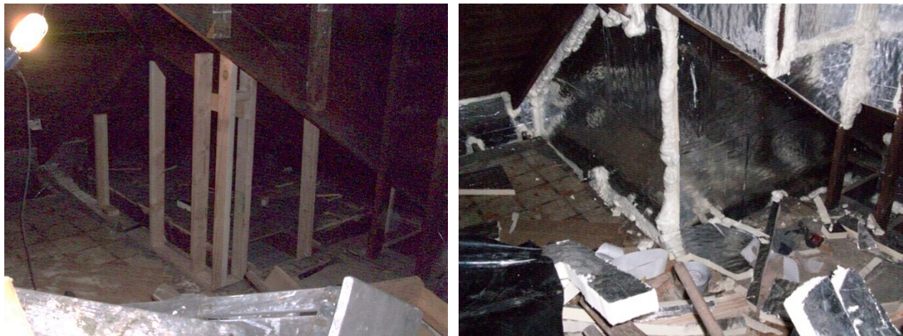
Figure 20. Left: Framing added above exterior wall at inset entry; Right: rigid board insulation installed to transition thermal control from exterior wall to roof assembly
