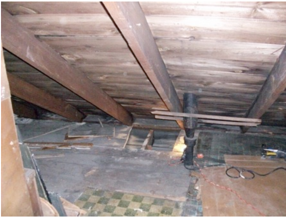
Figure 3. Left: Attic floorboards removed to investigate conditions at top of wall during assessment of prototype house; Right: Attic floorboards removed to allow access to top of wall
