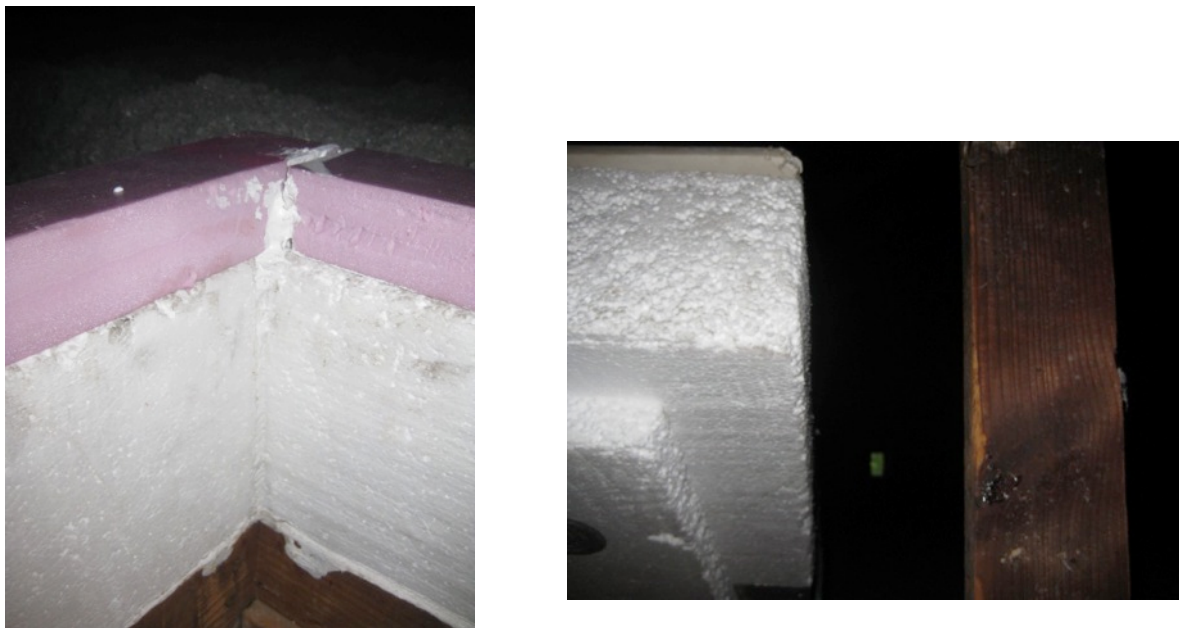
Figure 13. Left: Corner of attic access hatch insulation dam and frame; Right: Attic hatch insulated but without gaskets
