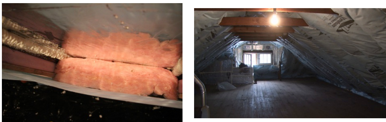
Figure 26. High density fiberglass batt in extended rafter cavity; Right: Completed roof rafter strategy (Photo credit: S. Marchese, printed with permission)
