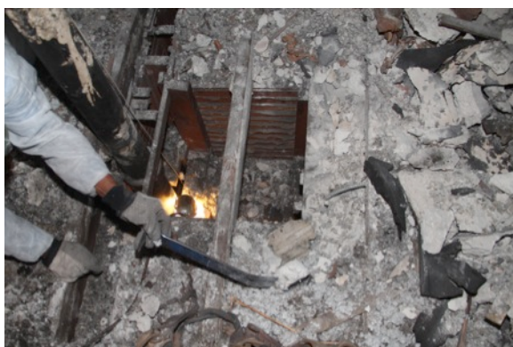
Figure 9. Left: Creating access to dropped soffit area and plumbing wall; Right: Attic floorboard repurposed in sealing plumbing chase (Photo credit: S. Marchese, printed with permission)
