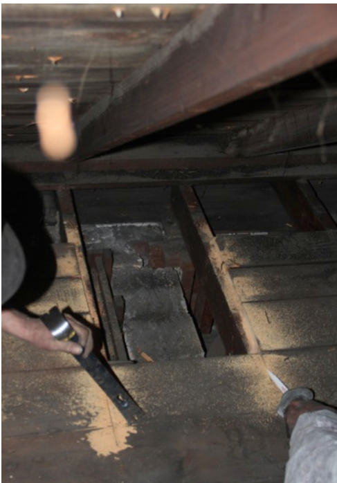
Figure 18. Left: Workers cutting access to expose top of exterior wall and furring cavity; Right: Access cut to expose top of exterior wall and furring cavity at inset opening (Photo credit: S. Marchese, printed with permission)
