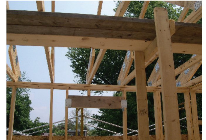
In-line trusses and wall studs @ 24" O.C. framing
