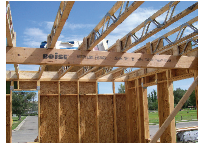
In-line open web floor joists and wall studs @ 24" O.C. framing
