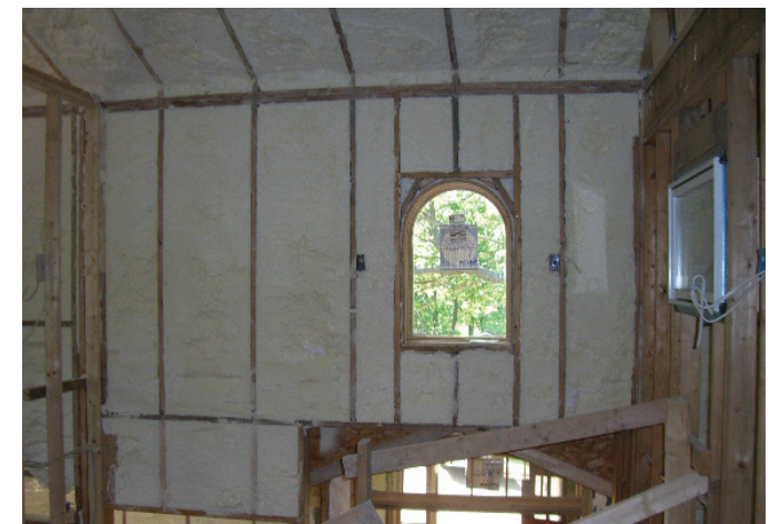
In-line rafters and wall studs @ 24" O.C. with cavity insulation
