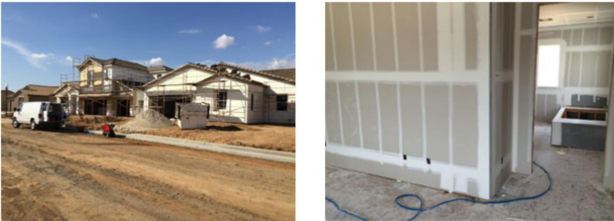
**Figure 1. Photo of housing development where the aerosol envelope sealing installations were performed and photo showing stage of construction the homes were in before sealing.**
