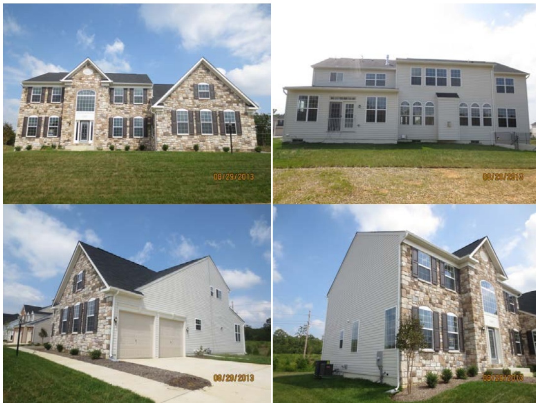
Figure 1. Top left: front view of the test house; top right: rear view; bottom left: front-right view; bottom-right: front left view
