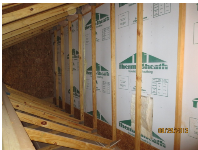
Figure 8. Back side of house-to-garage attic wall
